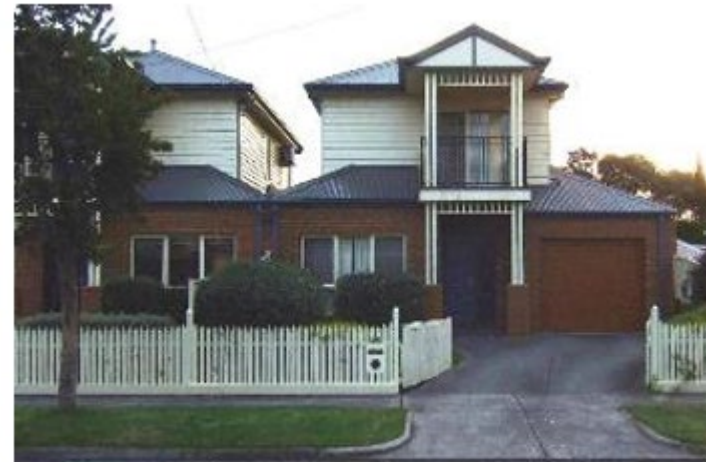
Design Controls are needed to guide development where the second floor has a smaller floorplate than the ground floor (sometimes known as 'pop-up').
