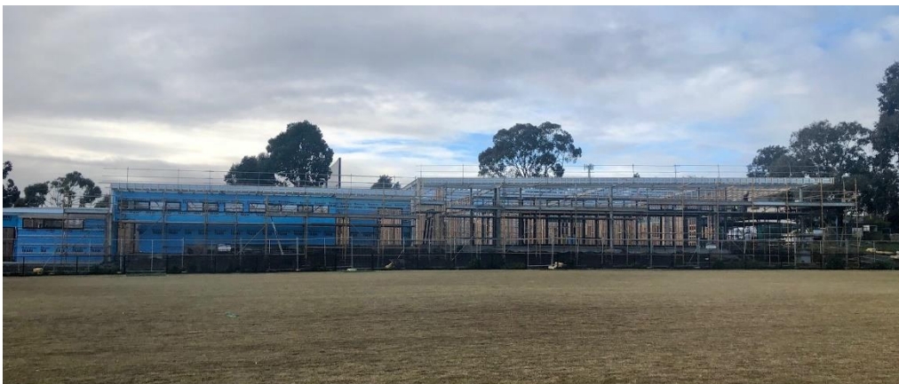
Figure 1: New pavilion at Donald McLean Reserve under construction
