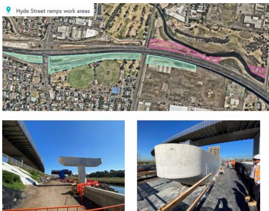
Figure 5: Hyde Street ramps – map of work areas and photos of construction
