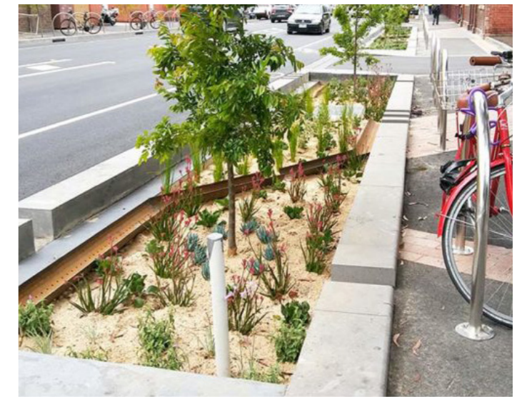
Example of a rain garden which contributes to the amenity of the street.
