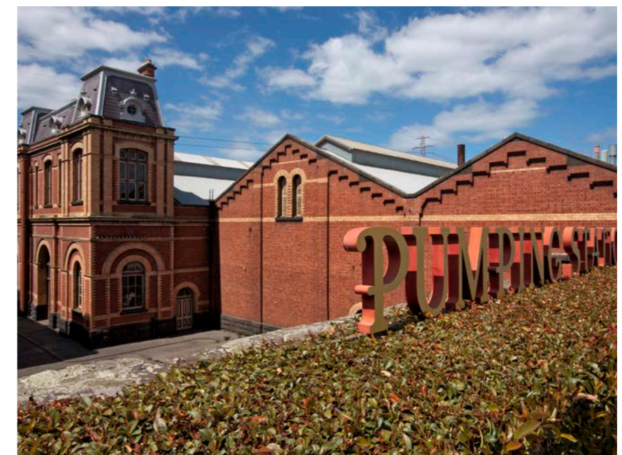
The Spotswood Pumping Station is an example of significant 19th Century industrial architecture that should be protected and celebrated.
