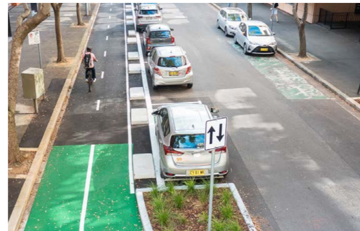
Example of an on road two way separated bike path (Source: City of Sydney)
