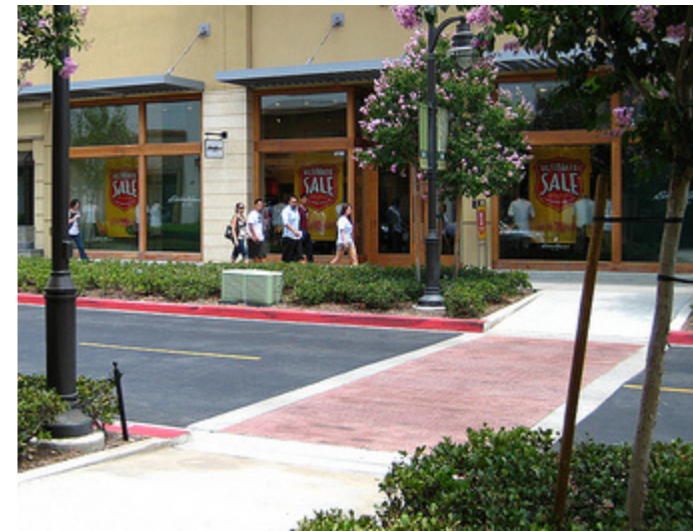
Example of a safe and comfortable crossing that allows for large vehicle movement.
