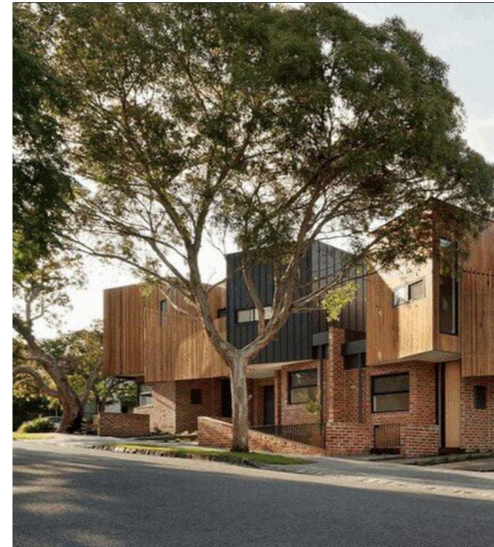
Example of an appropriate multi dwelling development (Source: Green Sheep Collective)
