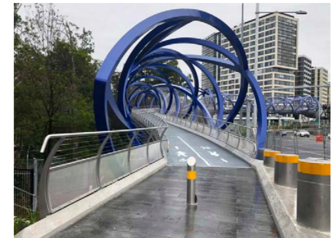
Grade separation is a potential solution for a safe pedestrian and cyclist crossing at the intersection of Craig Street and Douglas Parade (Source: The Urban Developer).
