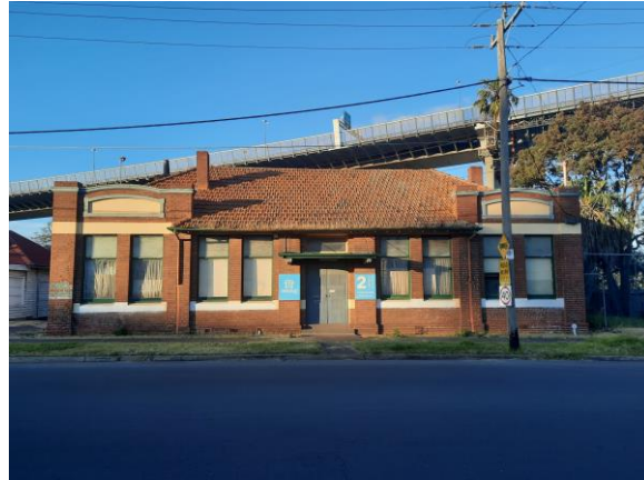
AGM Company Headquarters, Simcock Avenue
