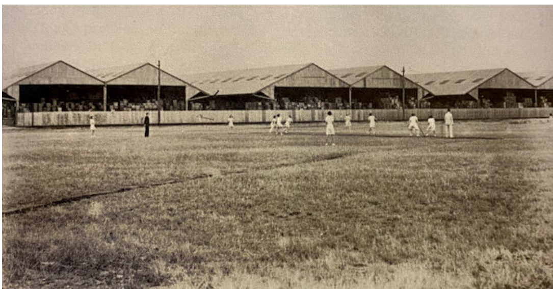
View to three of the corrugated sheds across Hudsons Road (west end), likely the late 1930s – prior to their concealment by the cream brick facades/buildings in the postwar period (Source: Tom Marshall Collection via Moloney, A history of the Melbourne Glass Bottle Works site )
