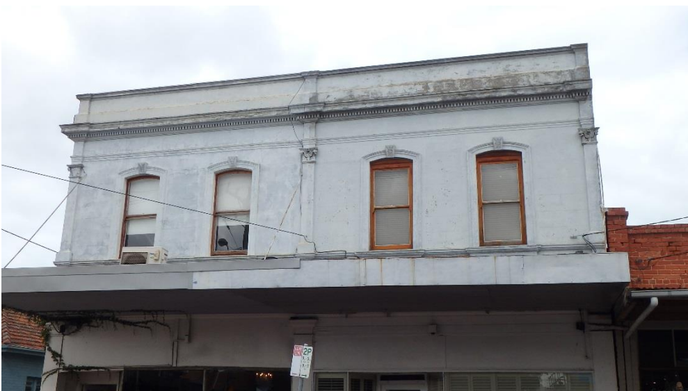
Upper part of Hudsons Road facade
