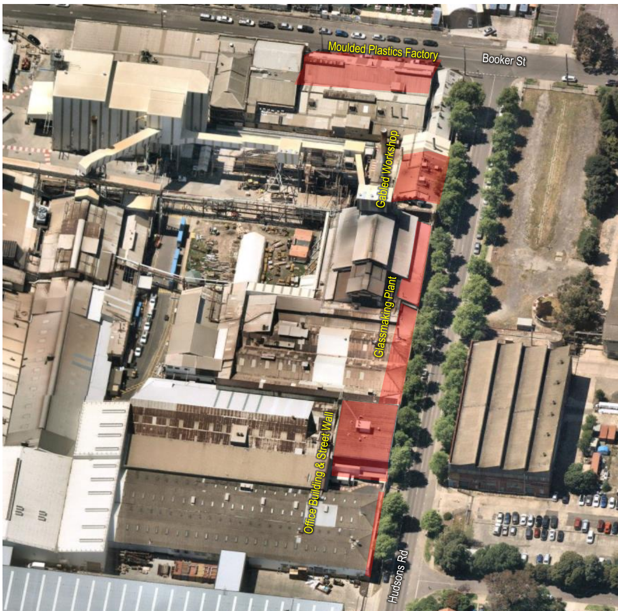
Aerial photograph of the Hudsons Road Buildings with significant fabric shaded red (Source: Nearmap, November 2020)
