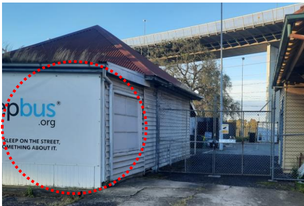
Tennis Clubhouse from Simcock Avenue (left), addition highlighted
