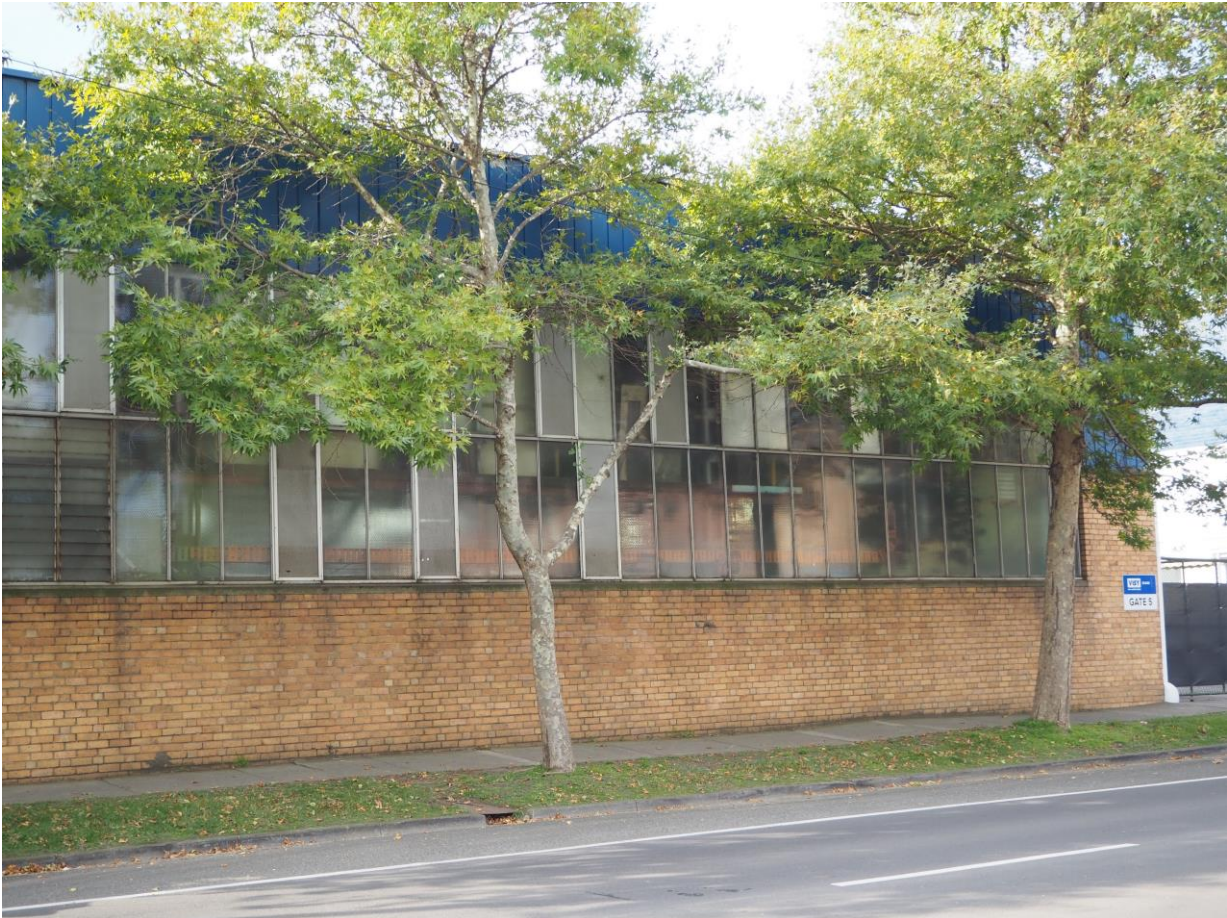
Postwar Street Wall, west of the entrance bay
