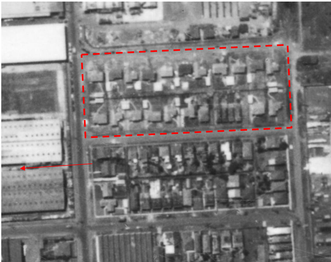
The estate in 1956 shortly after completion (north to left) (Source: Melbourne Outer Suburbs Project, Run 7, Frame 84, Landata)
