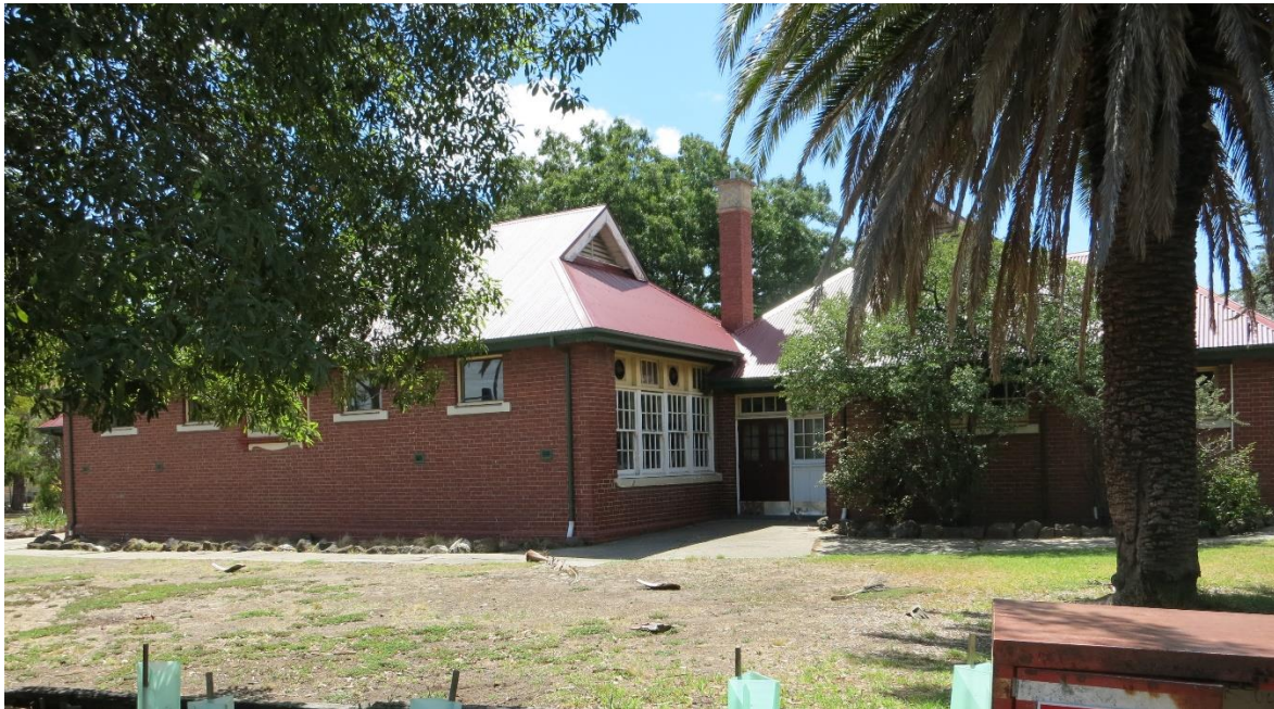
Intersection of western and southern wing of original section
