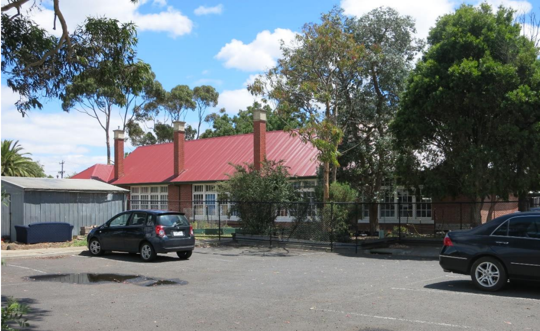
Southern wing. The rightmost bays are identifiable as the 1929 additions by the horizontal glazing bars to the toplight
