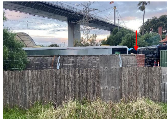
WWII Air Raid Shelter/Bunker , west elevation, brick end walls (arrow) with the parabolic concrete core behind
