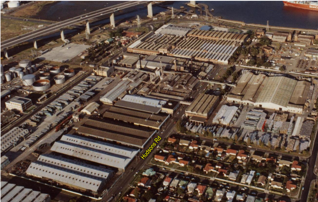
The ACI Complex, viewed from the west, 1979 (Source: Wolfgang Sievers, NLA, http://nla.gov.au/nla.obj-160330823 )
