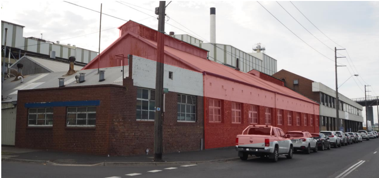
Moulded Plastics Building (significant part shaded red) viewed from the intersection of Hudsons Road and Booker Street
