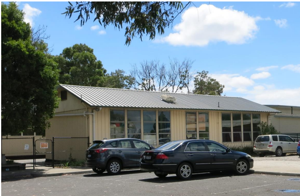
Double Bristol unit building facing McLister Street
