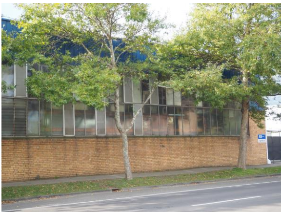
Street Wall, Hudsons Road (north)
