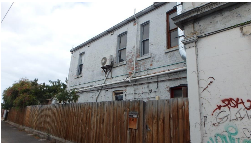
Rear wing (east elevation)
