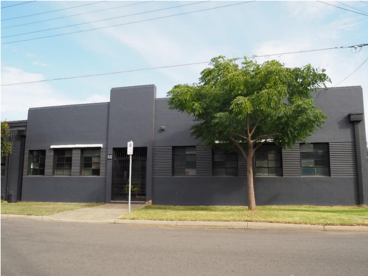
Craig Street façade – west end
