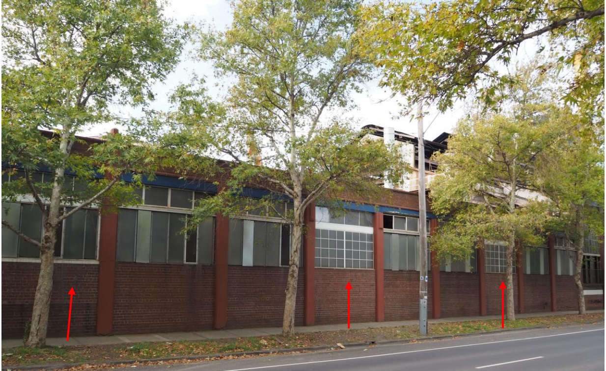
Single-storey section of the Glassmaking Plant , the original nine bays. Bays initially with roller doors highlighted
