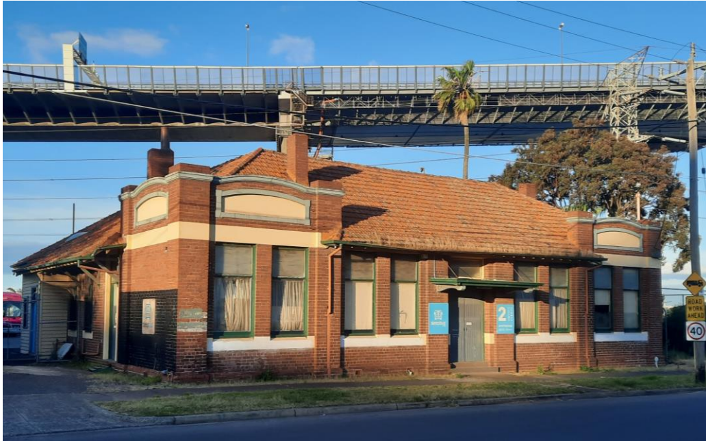
AGM Company Headquarters, Simcock Avenue frontage
