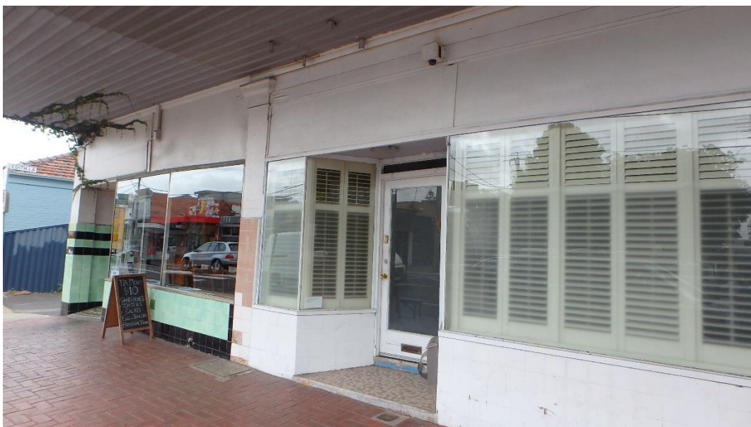
Shopfronts to Hudsons Road
