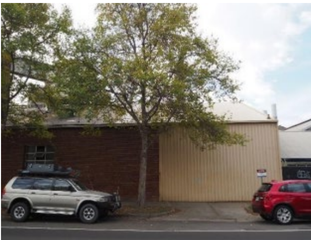
Figure 20 Metal clad extension to Gabled Workshop
