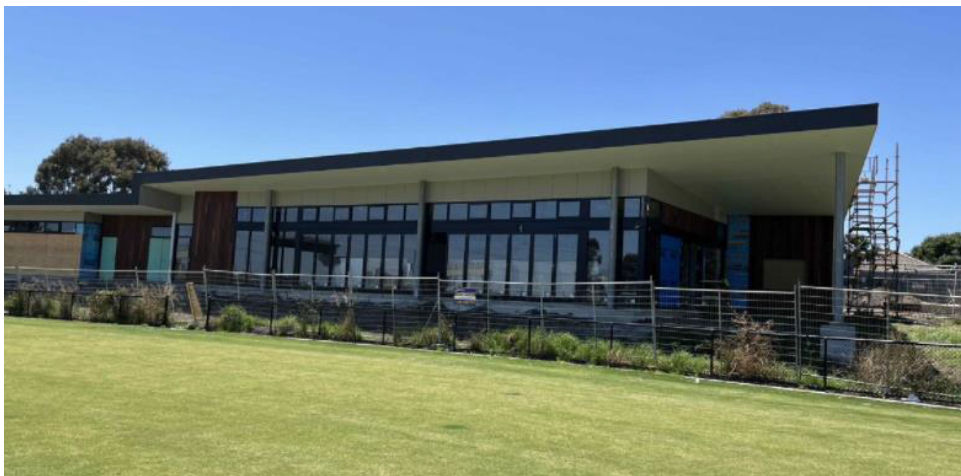
Figure 2: Couch Pavilion under construction at Donald McLean Reserve
