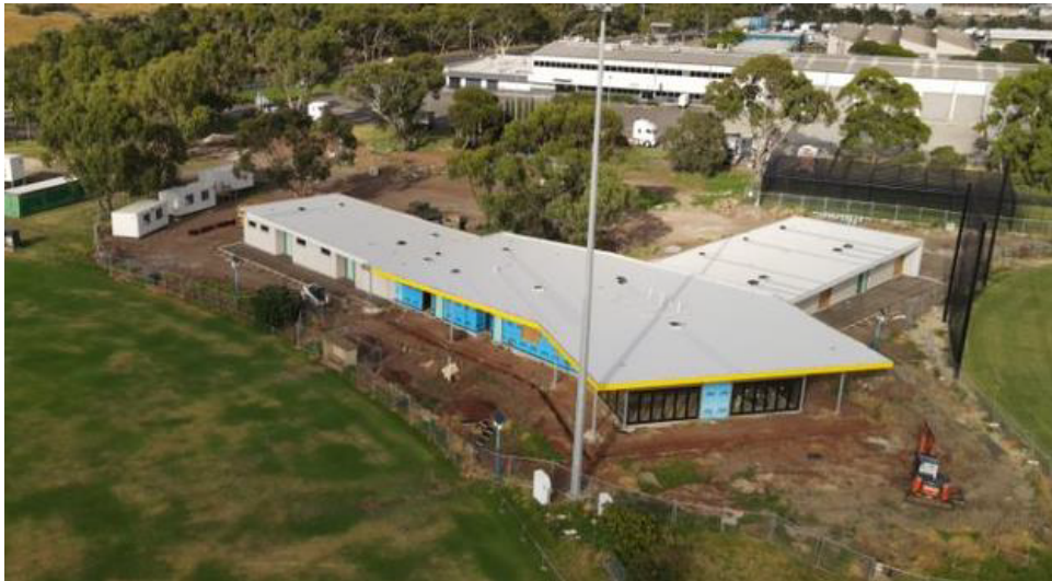
Figure 1: WLJ Crofts Reserve pavilion under construction
