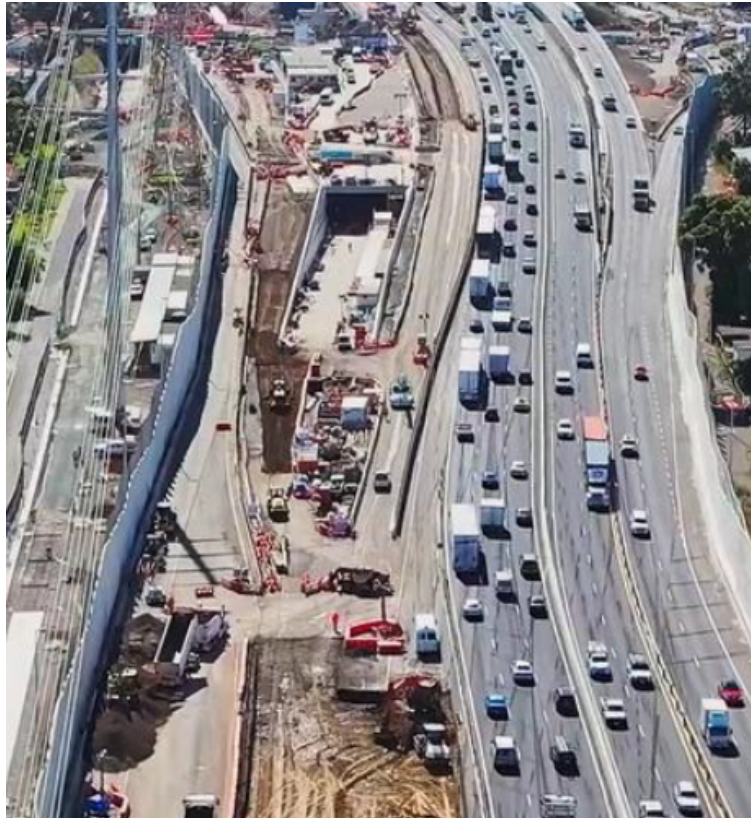
Figure 4: Traffic switch around inbound tunnel portal works
