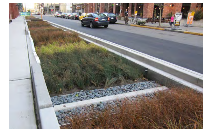
Rain garden and new trees on kerb extension. First road narrowing to 'mark the entry' to the precinct
