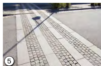
Ballast stone and dark sawn bluestone in carriageway ramps and pedestrian crossing
