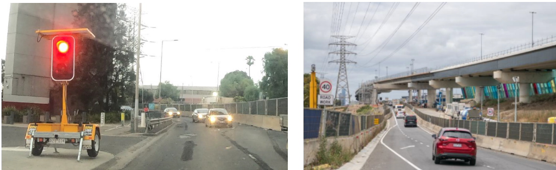
Figure 6: Hyde Street shuttle traffic flow and ramp construction
