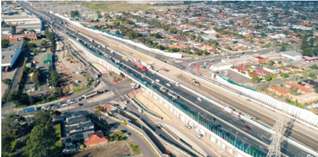
Figure 2: Works at Millers Road
