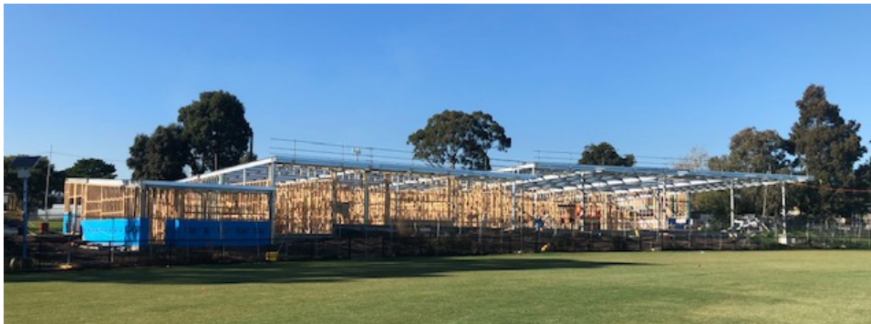
Figure 2: WH Couch Pavilion under construction
