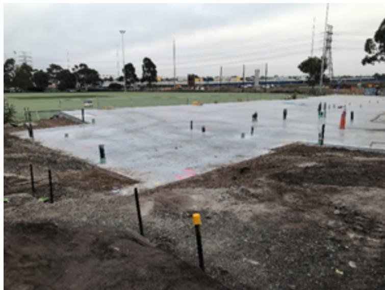
Figure 4: Concrete slab for the new WH Couch Pavilion at Donald McLean Reserve
