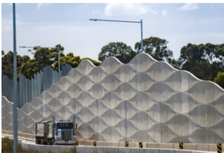
Figure 2: Newly installed noise walls at the Millers Road outbound on-ramp
