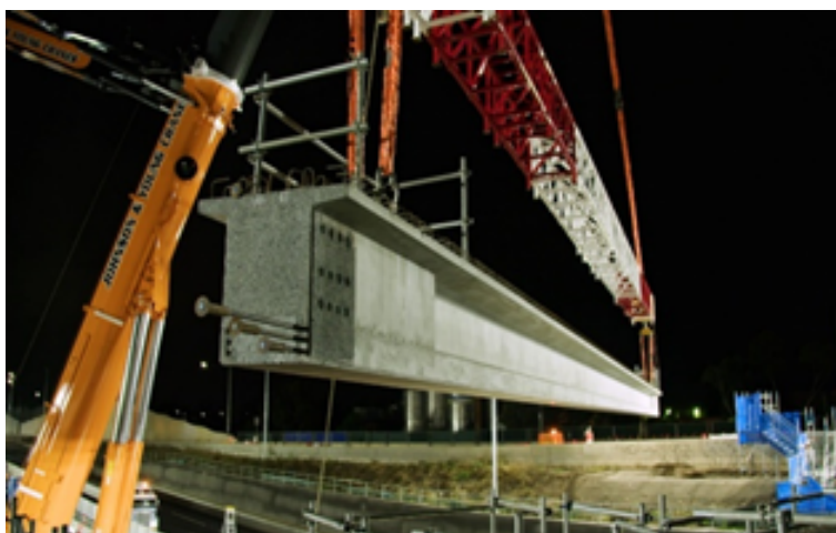
Figure 1: Grieve Parade bridge works over the freeway
