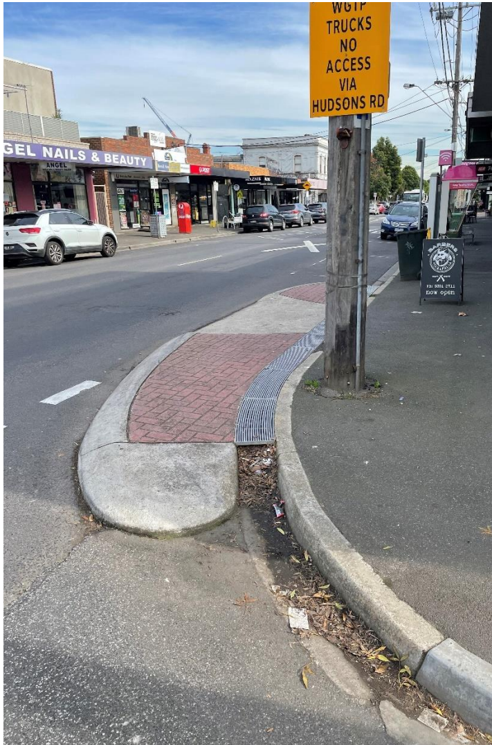
Figure 10 Current Raised Pavement Arrangement
