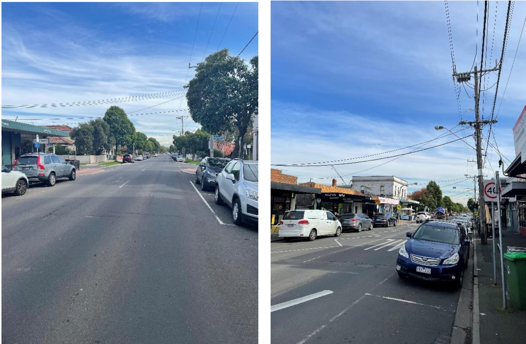
Figure 4 Overhead Powerlines with minimal clearance
