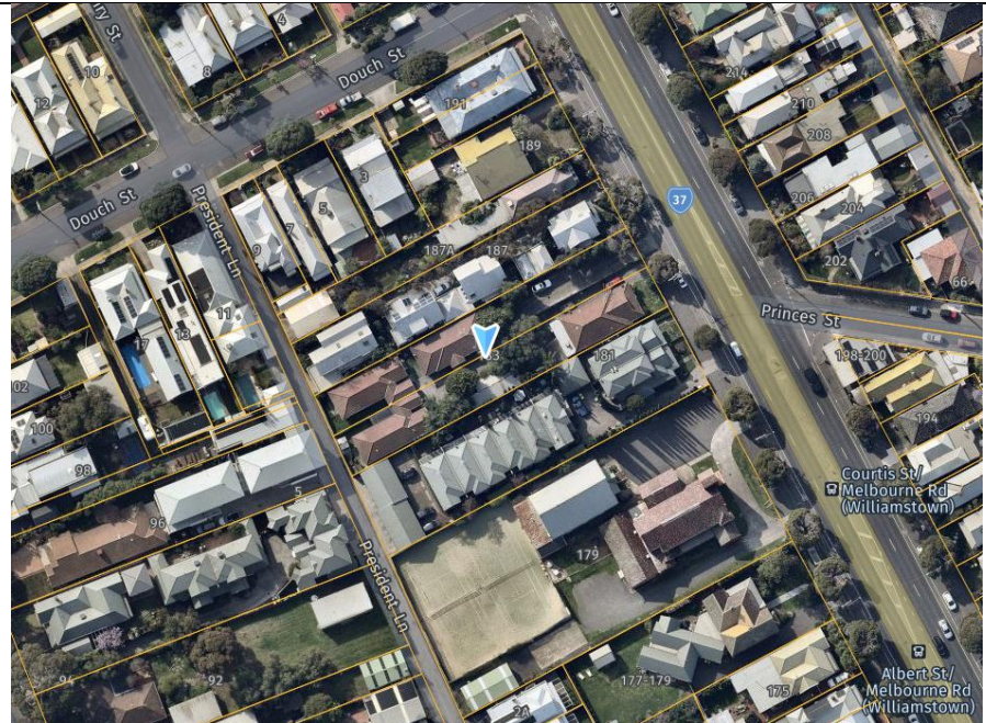
Arial photo of 183 & 185 Melbourne Road and the surrounding area.
