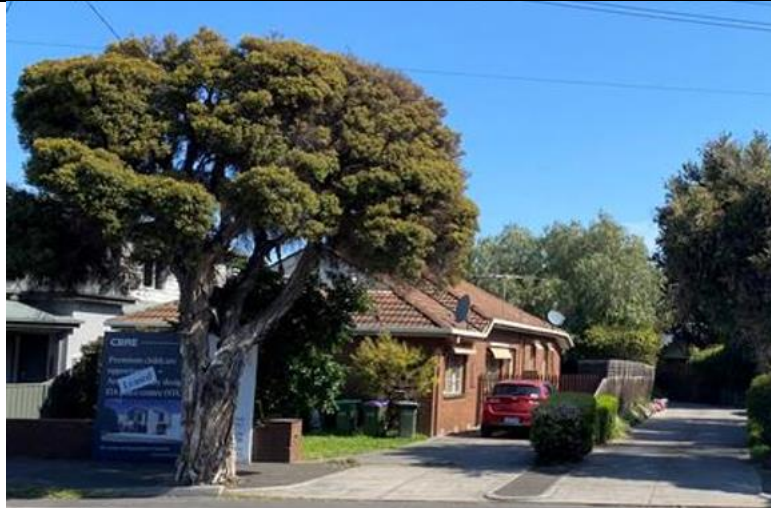
From across the road facing south-west
