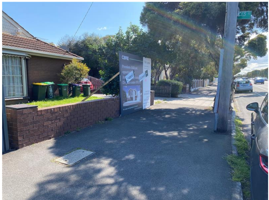
183 Melbourne Road from the footpath facing north-west
