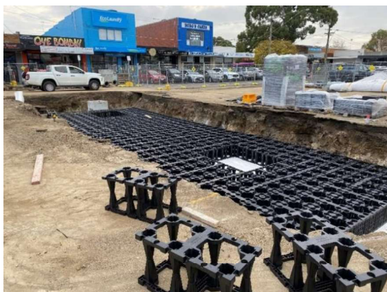
Image: New strata tree cells installed at Harrington Square for better root growth of new trees
