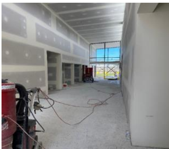
Image: Dennis Reserve, main building corridor
