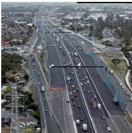
Image: West Zone completions – West Gate Freeway, Millers Road
