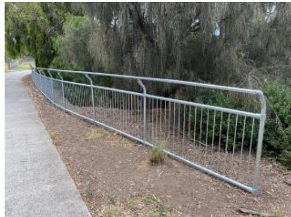
Image: Kororoit Creek Shared Pathway
