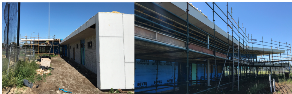
Figure 1: WLJ Crofts Reserve pavilion under construction
