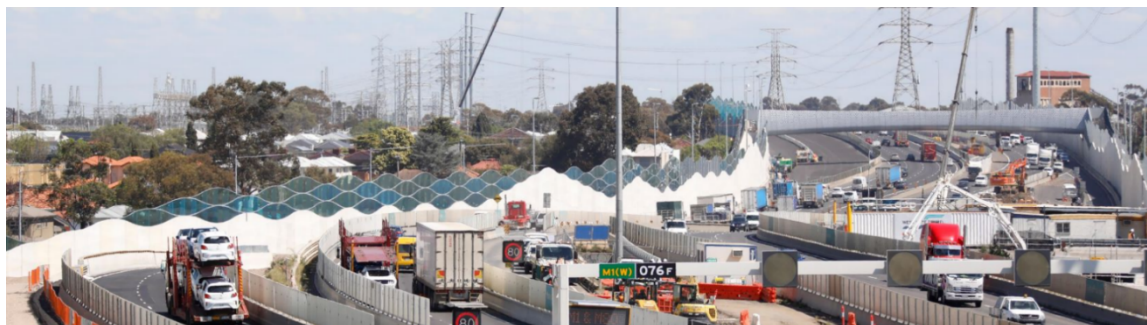
Figure 3: Looking west towards Muir Road pedestrian overpass
