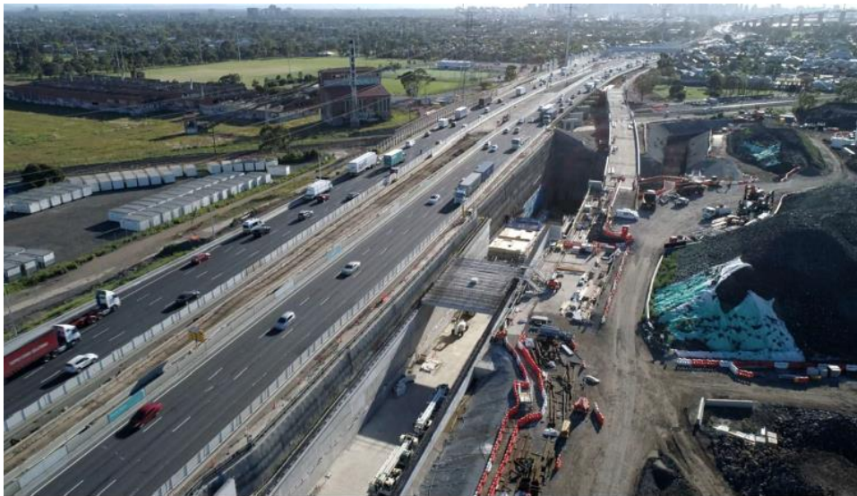
Figure 9: Southern Outbound Tunnel Portal
