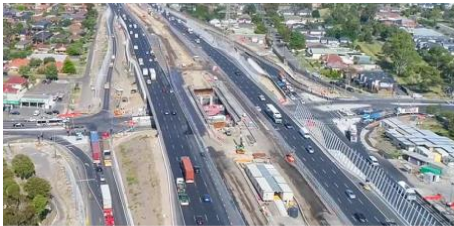
Figure 6: Millers Road interchange works
