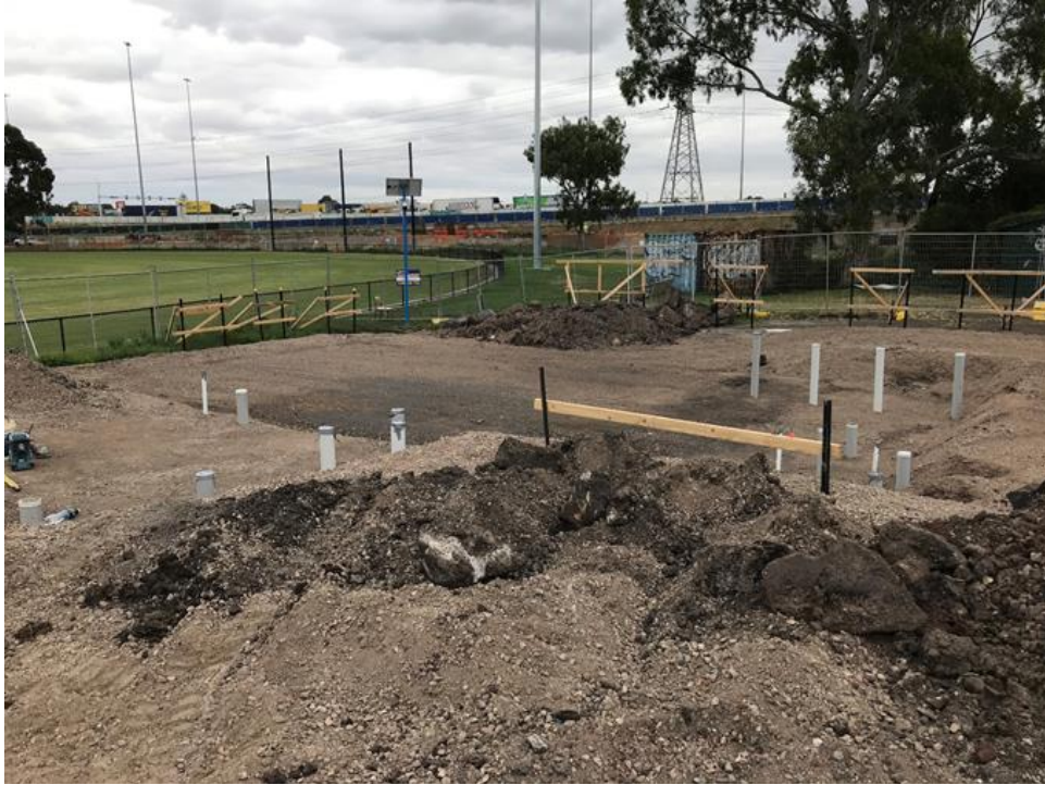
Figure 2: Foundation works for the new pavilion at Donald McLean Reserve
