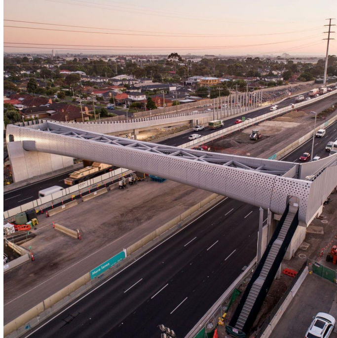
Figure 8: New Pedestrian Overpass
