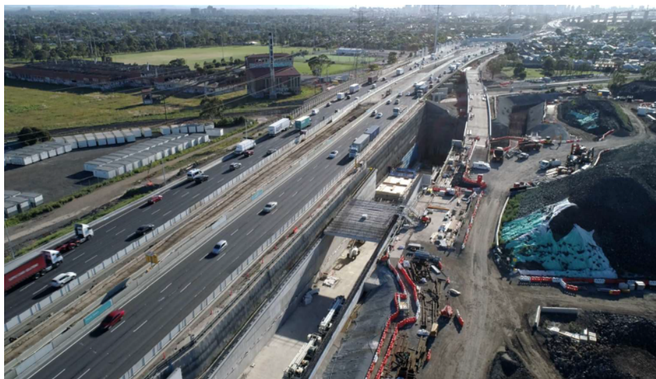
Figure 9: Southern Outbound Tunnel Portal
