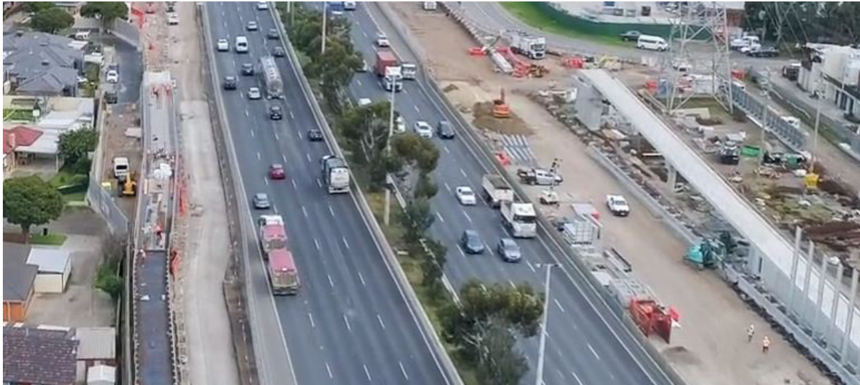
Figure 1: Rosala Avenue pedestrian overpass construction
