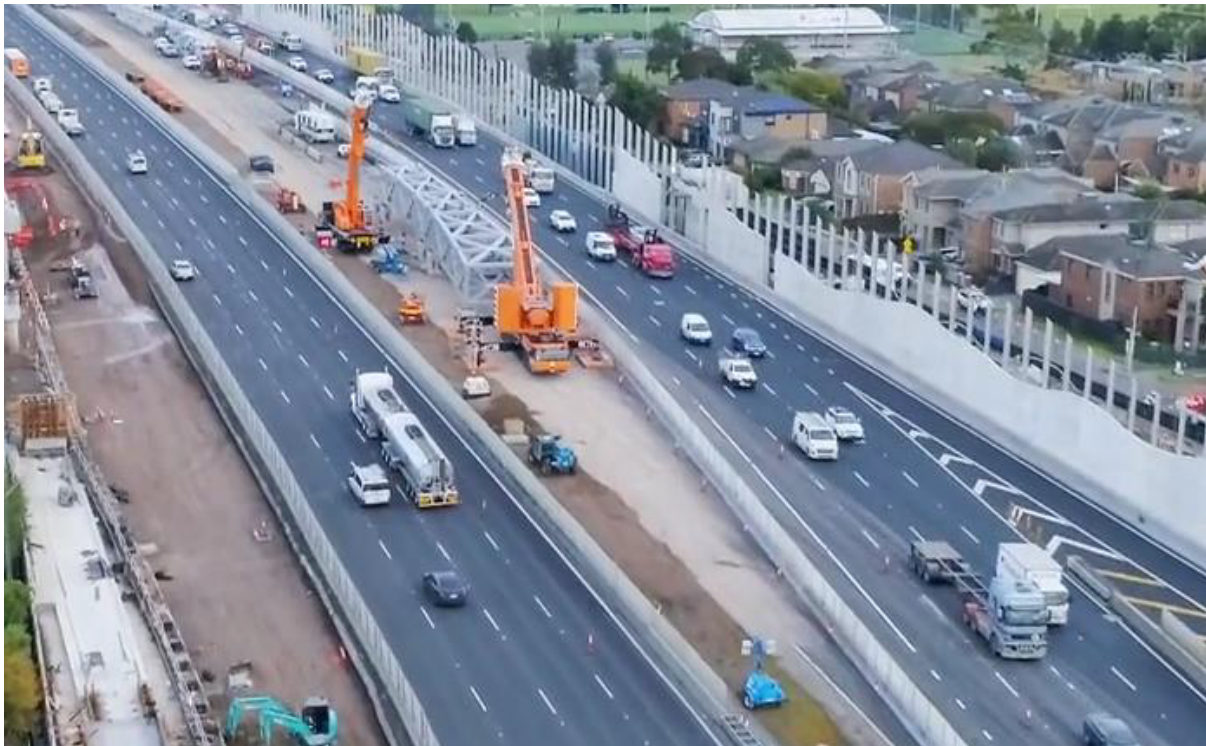
Figure 2: Muir Street pedestrian overpass construction
