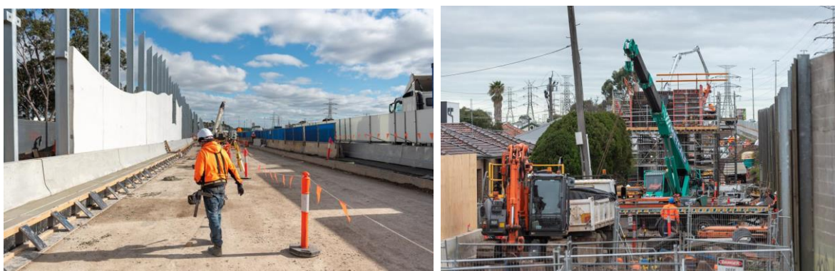
Figure 2: WGTP works along the freeway
