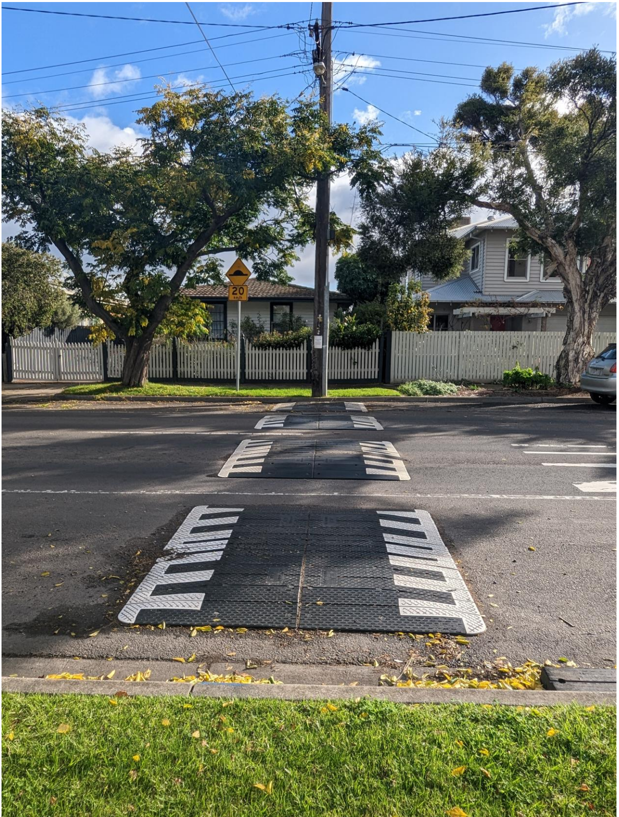
Source: Photo taken during site inspection of existing speed cushions on Maddox Road
