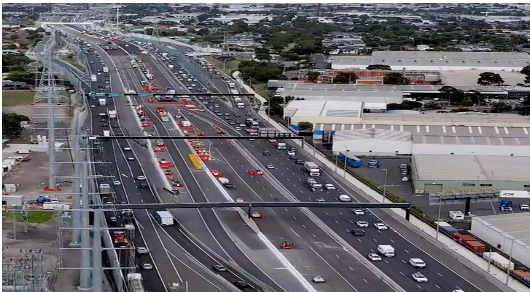
Figure 2: West Gate Freeway West Zone works – outbound
