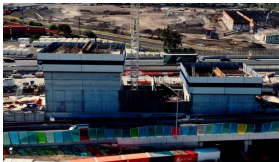
Image: Southern Outbound Portal Vent Structure under construction
