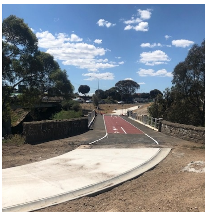
Figure 1: New SUP over Kororoit Creek
