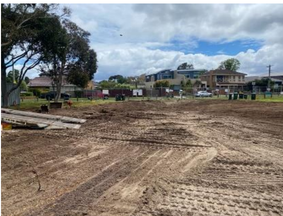
Image: Site following the demolition of Seaholme Kindergarten
