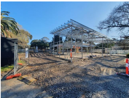
Image: Dennis Reserve, new structure (western side)
