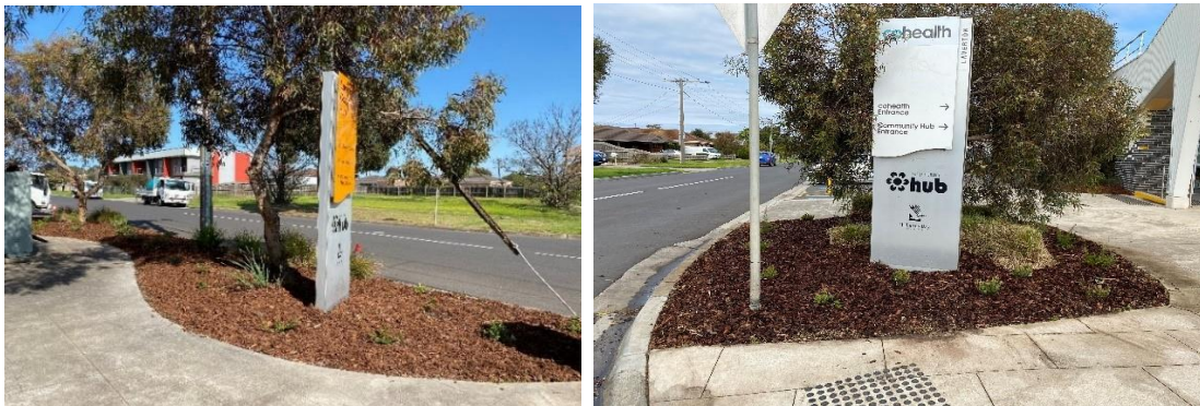
Image: Laverton Hub completed works
