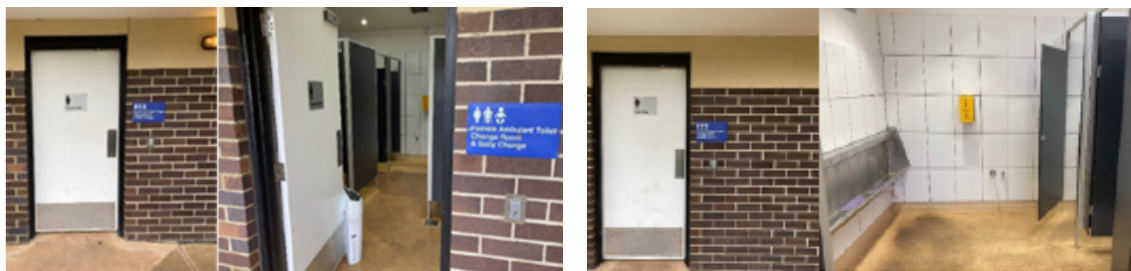
Figure 1: Weaver Reserve public toilets with signage showing female symbols and internal space with cubicles (left), and with signage showing male symbols and internal space with urinals and cubicles (right)
