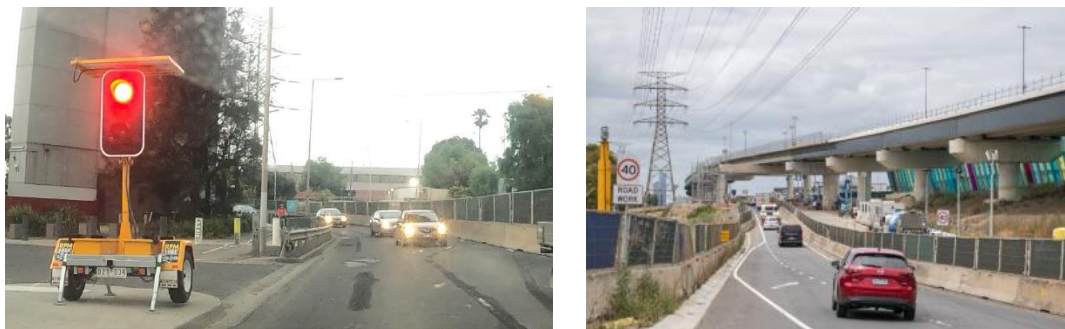
Figure 6: Hyde Street shuttle traffic flow and ramp construction
