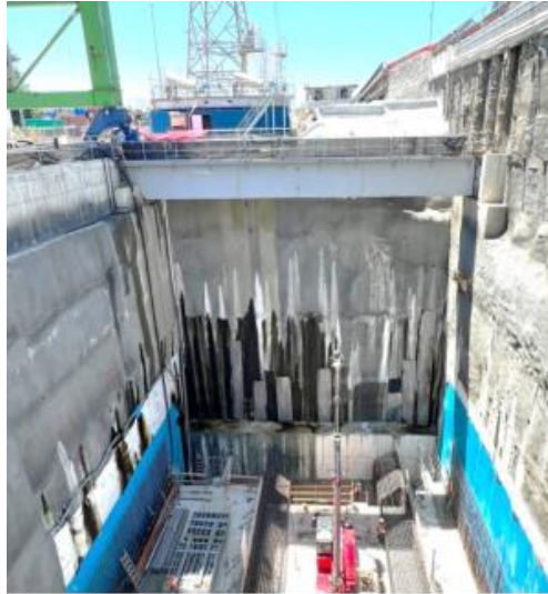
Figure 8: Headwall at southern inbound portal and concrete cradle in the 30m deep retrieval pit
