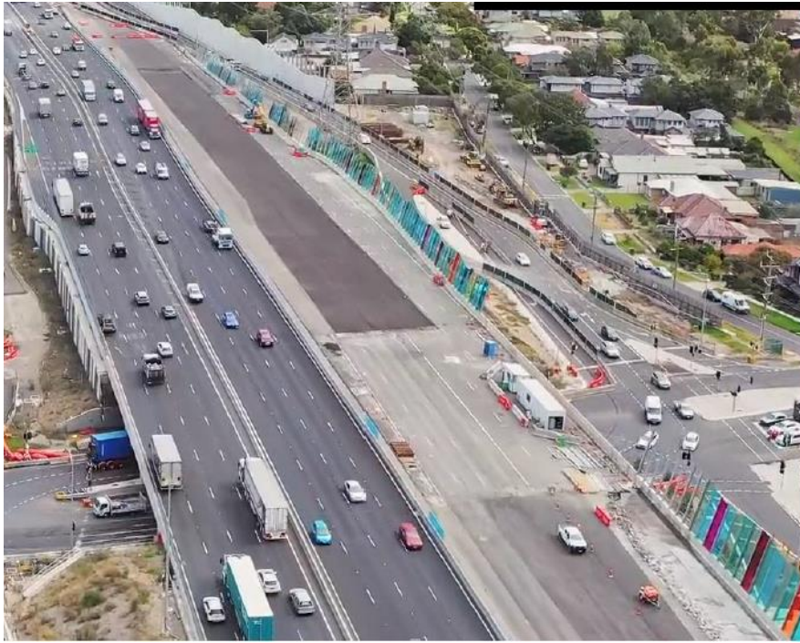
Figure 2: Works at Millers Road
