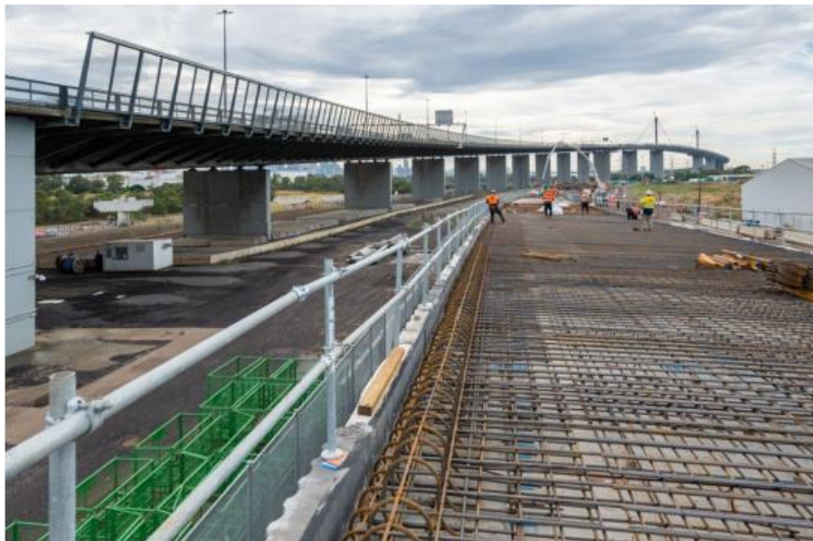
Figure 3: Hyde Street ramp works
