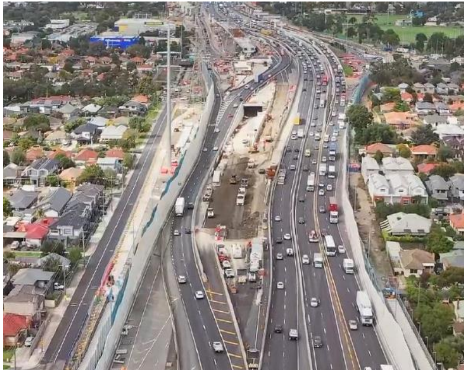
Figure 1: Traffic switch around inbound tunnel portal works
