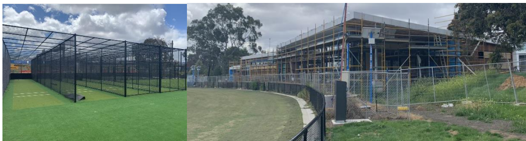
Figure 2: New cricket nets and WH Couch Pavilion under construction
