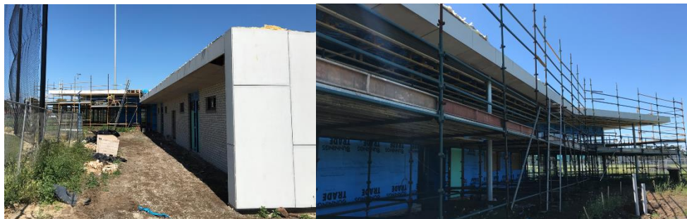
Figure 1: WLJ Crofts Reserve pavilion under construction
