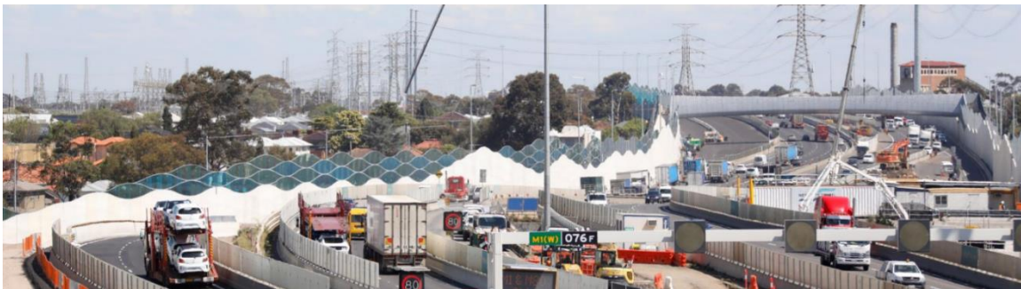
Figure 3: Looking west towards Muir Road pedestrian overpass
