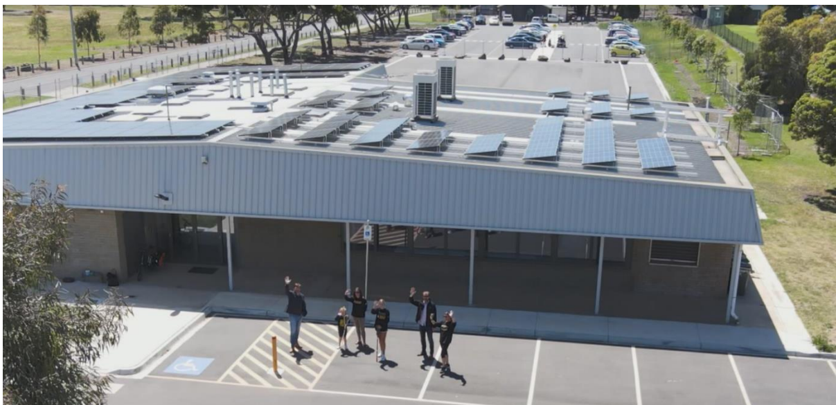
Figure 1: Celebrating the installation of the solar infrastructure at the Altona Lacrosse Pavilion
