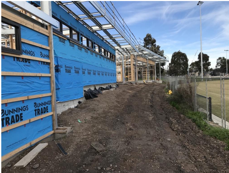
Figure 2: WH Couch Pavilion under construction
