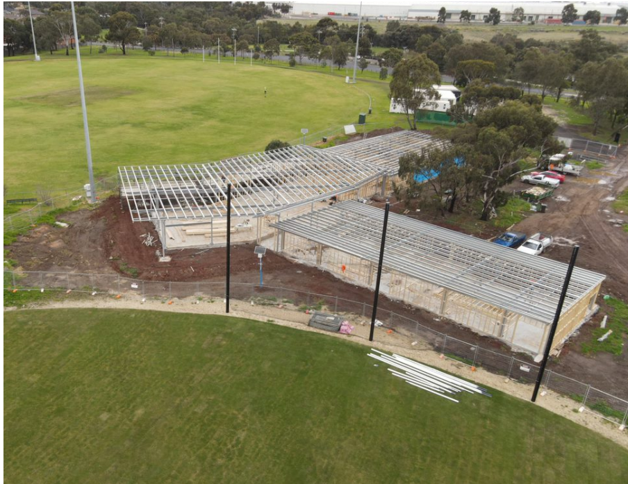
Figure 1: New pavilion at WLJ Crofts Reserve under construction
