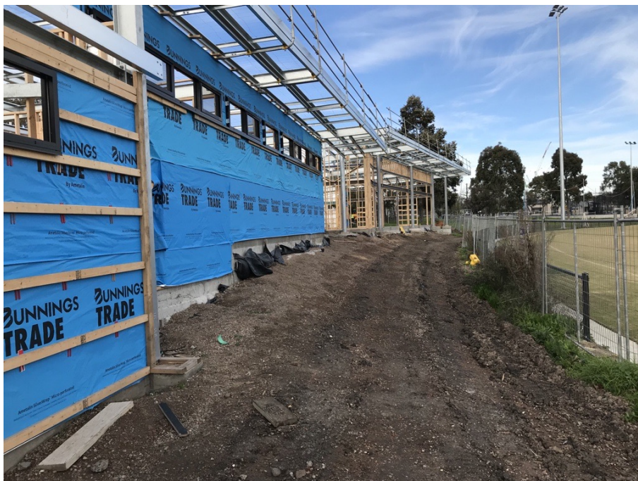
Figure 2: WH Couch Pavilion under construction
