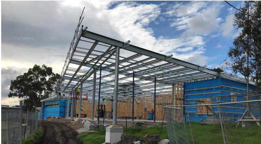
Figure 2: WH Couch Pavilion under construction
