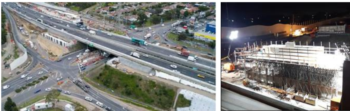
Figure 5: Works at Melbourne Road interchange
