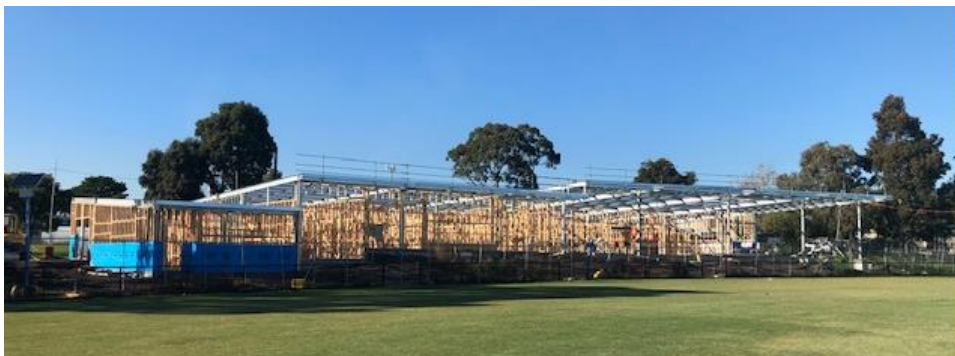
Figure 2: WH Couch Pavilion under construction
