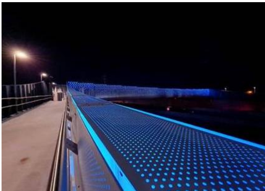
Figure 5: Pedestrian bridge images
