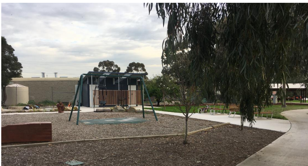
Figure 5: Brooklyn Reserve, Brooklyn – new public toilet close to the playground
