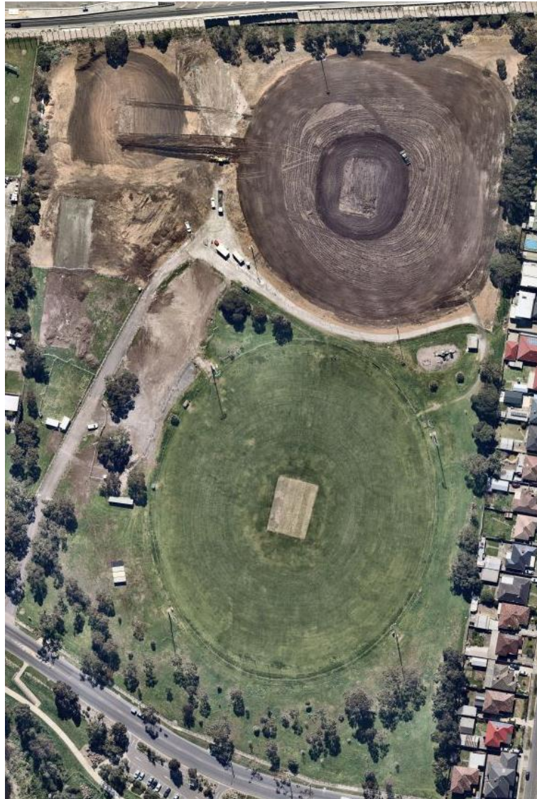
Figure 4: WLJ Crofts Reserve, Altona North – demolished pavilion and earthworks
