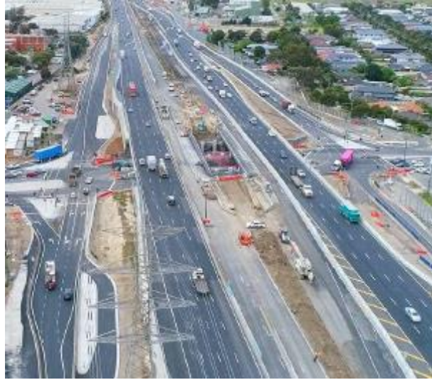
Figure 2: Millers Road interchange works
