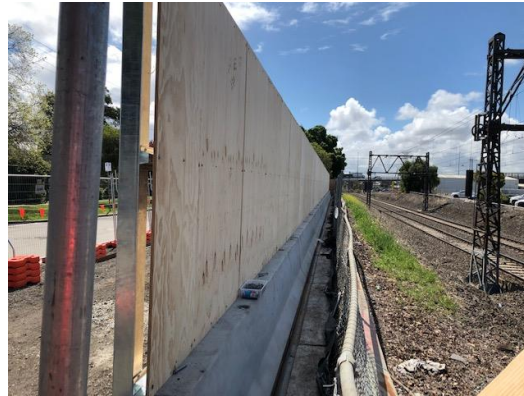
Figure 3: New temporary noise wall in Hope Street, Spotswood
