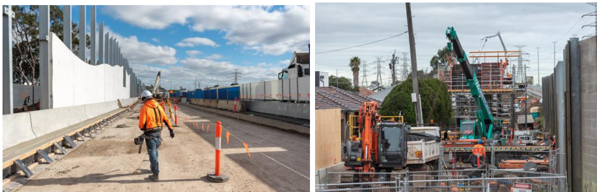
Figure 2: WGTP works along the freeway
