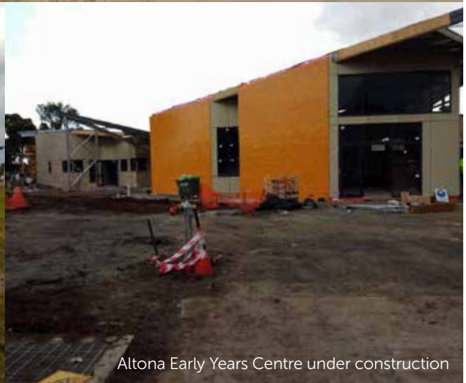
Altona Early Years Centre under construction
