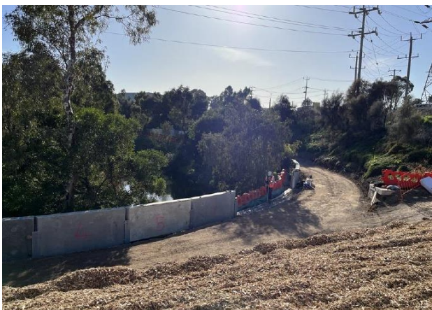
Image: Construction of the Kororoit Creek shared path
