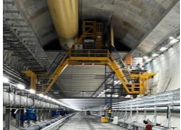
Image: Tunnel fitout underway
