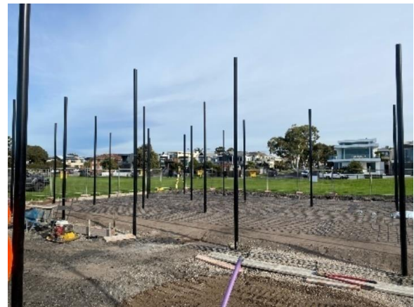
Image: Installation of new posts at Greenwich Reserve
