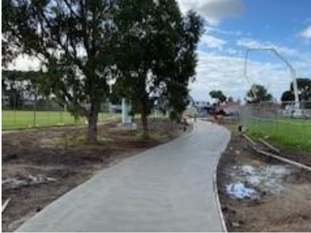
Image: Pathway works (pavilion to playground)
