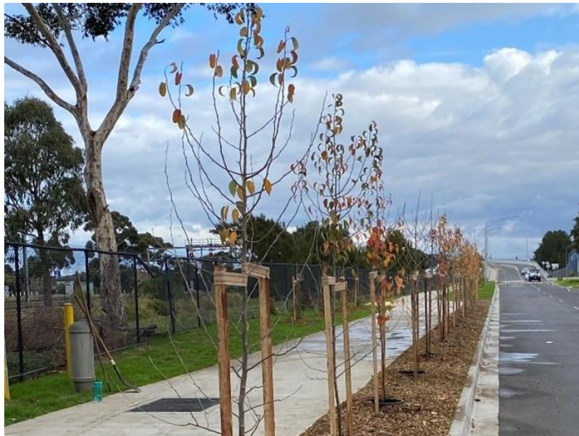
Image: Newly completed Maher Road Laverton, Shared User Path (May 2023)
