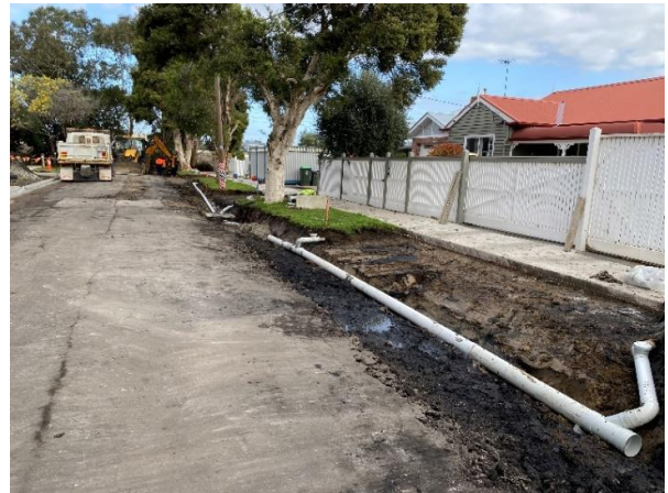
Image: Connection of drains along Port Street
