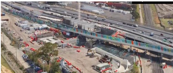
Image: Southern tunnel portal works
