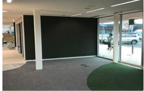
Image: Childrens room acoustic panelling being installed
