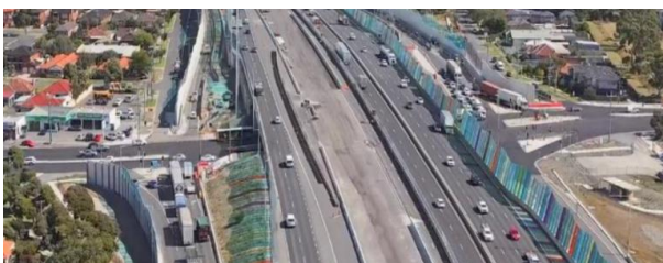
Image: Millers Road works completion
