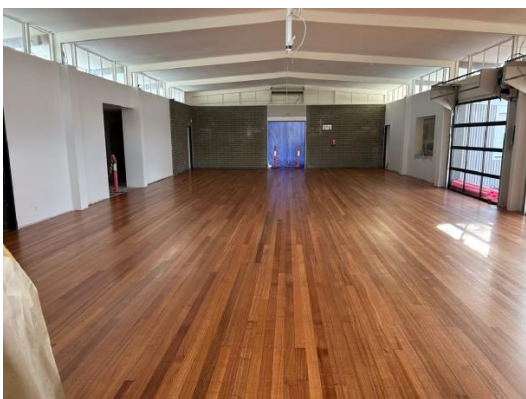
Image: Rejuvenated floorboards in the existing hall
