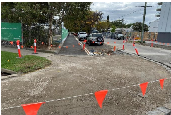
Image: Footpath at the intersection of Cecil and Kanowna Streets ready for asphalt
