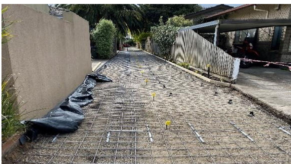
Image: Steel reinforcement being laid in Joiner Lane
