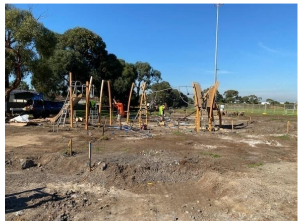
Image: Playground construction at WLJ Crofts Reserve
