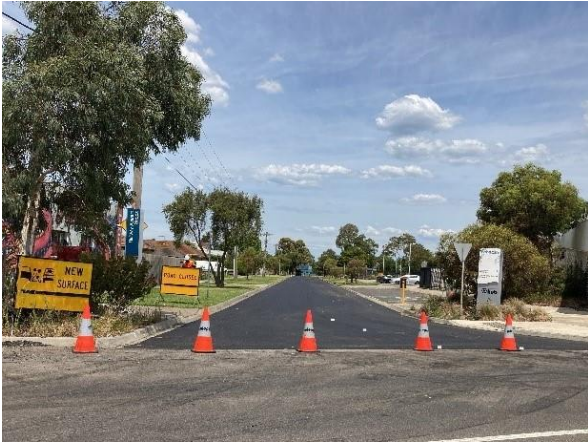
Image: Asphalt pavement just laid at Donald Street
