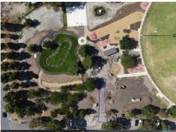
Image: Aerial photo of Donald McLean Reserve. The area marked out in blue shows the location of the concrete path. These works are currently underway
