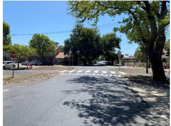
Image: New raised crossing at the intersection of Cecil and Parker Streets
