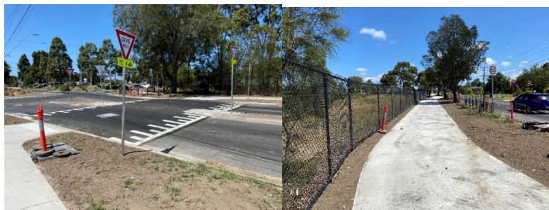
Images: Maher Road, Laverton – raised crossing near the intersection of Bladin Street and the shared path along Maher Road. This project was identified in the Place Guide
