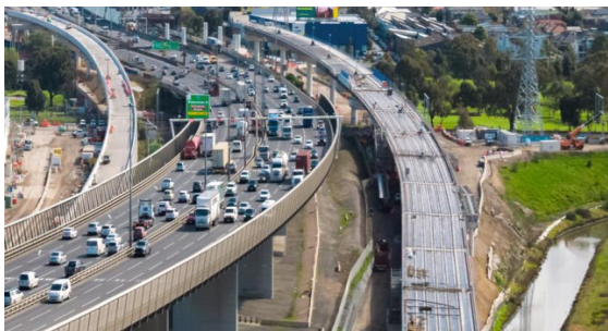
Above: New Hyde Street ramps under construction
