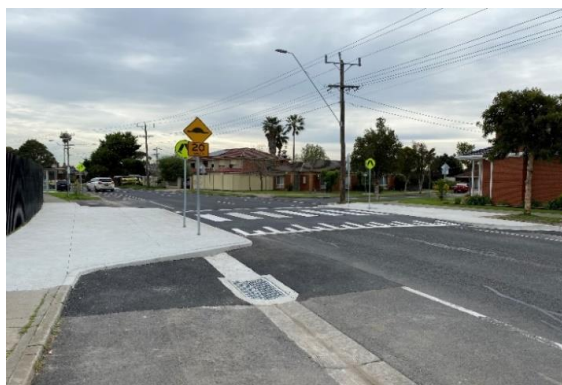
Above: New raised zebra crossing in Victoria Street
