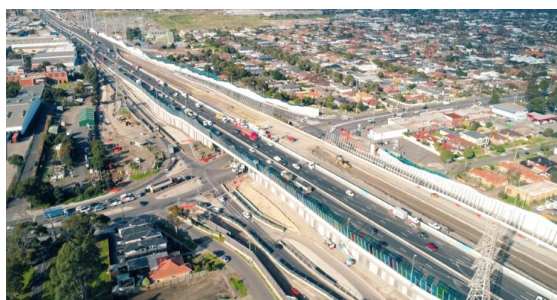
Above: Millers Road works
