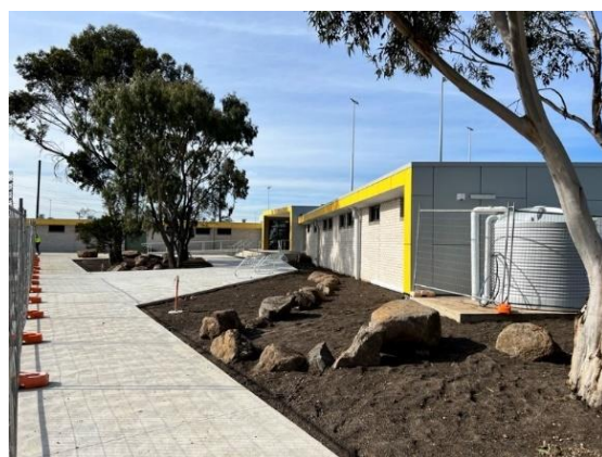
Above: Pavilion at Crofts Reserve
