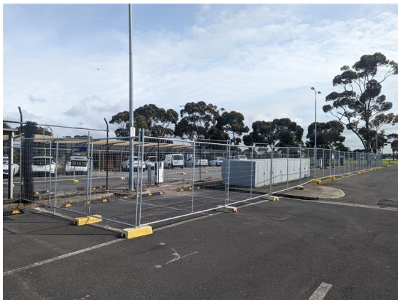
Above: Works at Hobsons Bay Civic Centre
