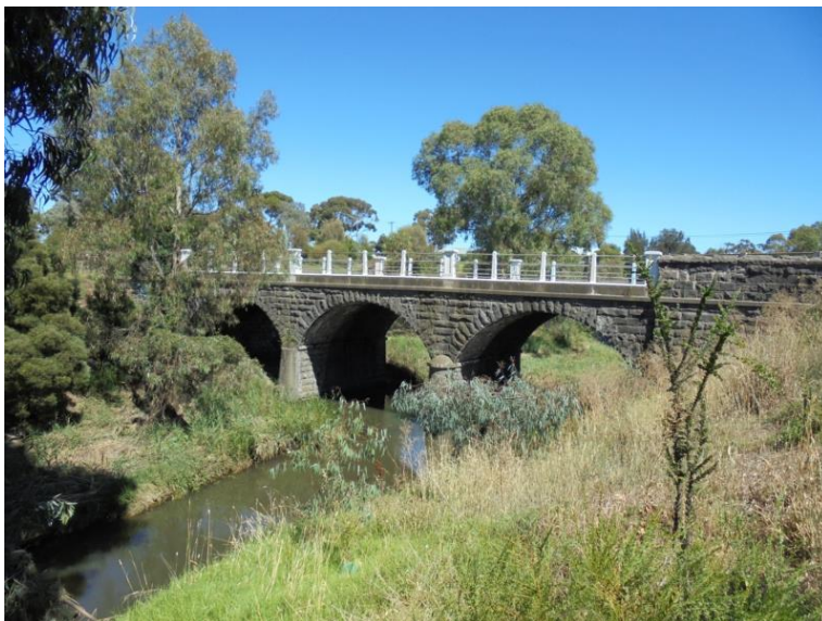
Above: Former Princes Highway bluestone bridge over Kororoit Creek, Brooklyn
