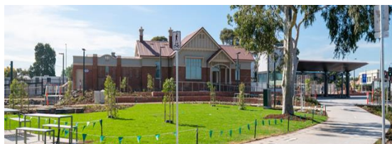
Above: The new North Williamstown station
