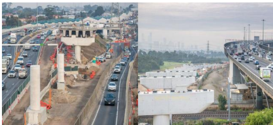
Above: Ongoing works on the Hyde Street ramps in Spotswood
