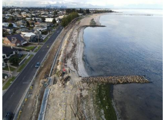
Above: Aerial image of the seawall works
