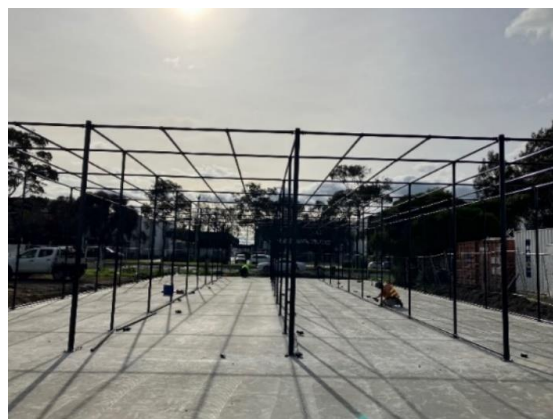
Above: Completed slab works at JT Gray
