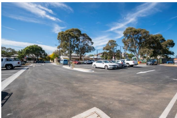
Above: the new North Williamstown station car park
