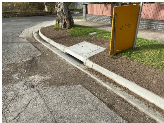
Above: Stage 2 drainage works completed in Aloha Street
