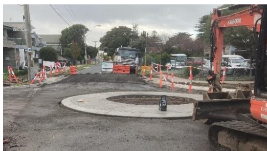
Above: Roundabout construction at Queen Street Altona
