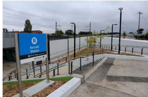
Above: New underpass at Aircraft station
