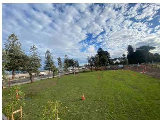
Above: Before and after turf installation at Weaver Reserve
