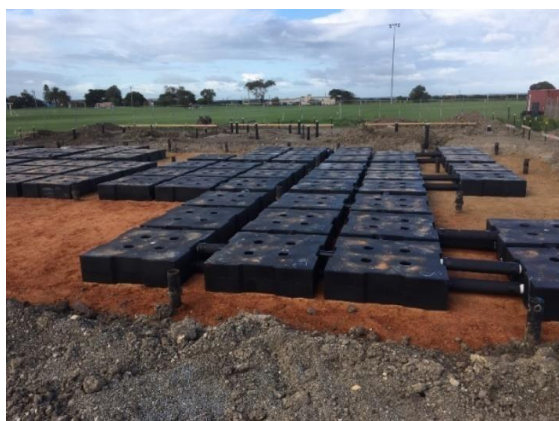
Above: installation of the under-slab water tanks
