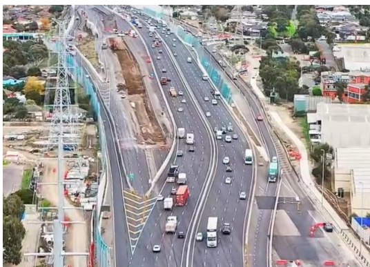
Above: Traffic switch on West Gate Freeway at Millers Road interchange
