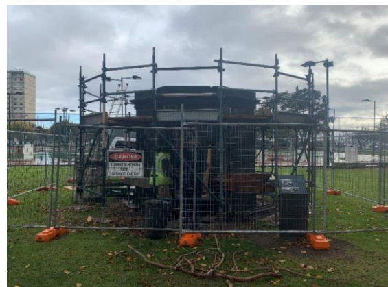
Above: Works at Tide Gauge House
