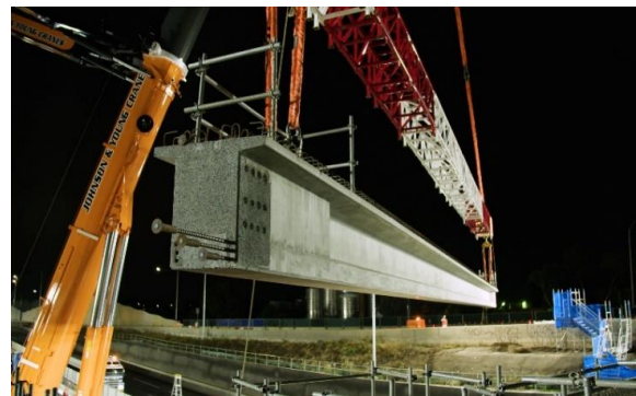
Above: Grieve Parade bridge works over the West Gate freeway
