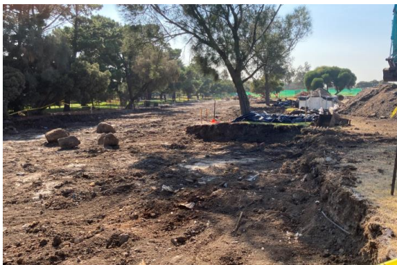
Above: Excavation works at PA Burns Reserve
