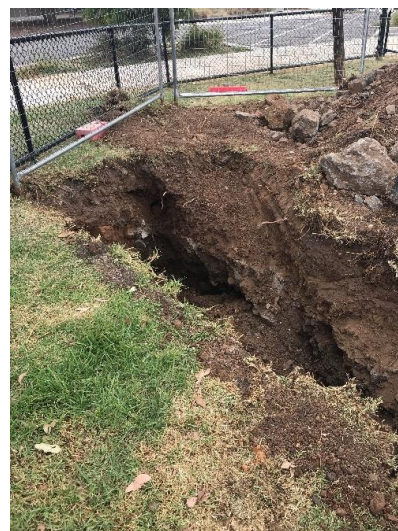
Above: Installation of electrical conduit at Bruce Comben
