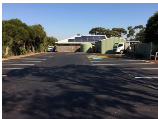
Above: Upgraded car park at the Altona North Lawn Bowls
