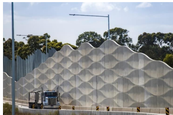
Above: Newly installed noise walls along Grieve Parade outbound exit ramp
