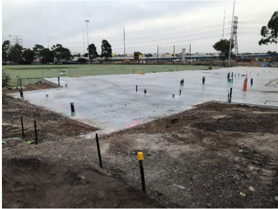
Above: Concrete slab works at Donald McLean
