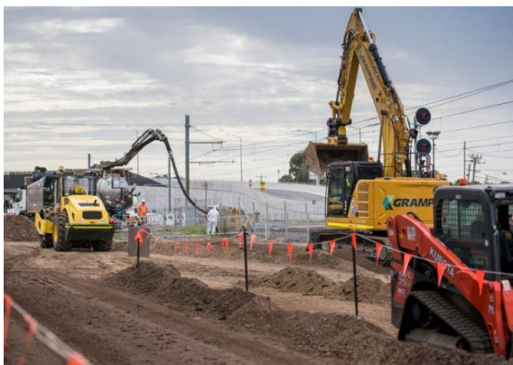
Above: Construction works at Aircraft Station
