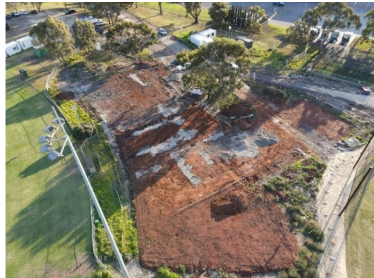
Above: Pavilion works at WLJ Crofts Reserve
