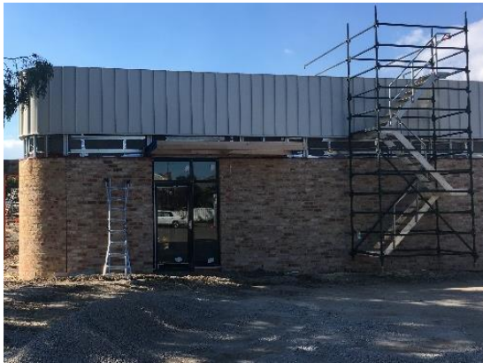
Above: Recycled chimney bricks for the south building
