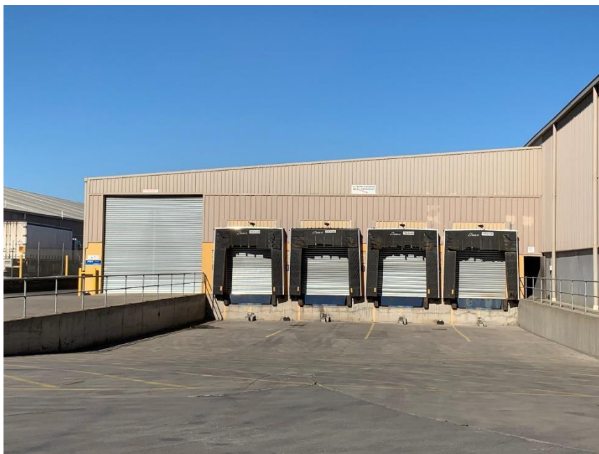
Figure 4 – Doors 3, 4, 5 and 6 and Door 7 to the far left
