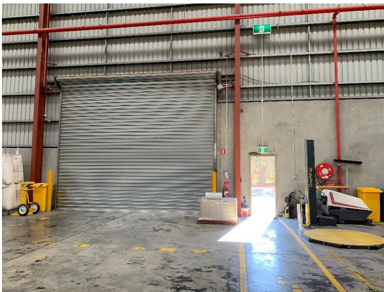
Figure 2 - Internal view of Door 1
