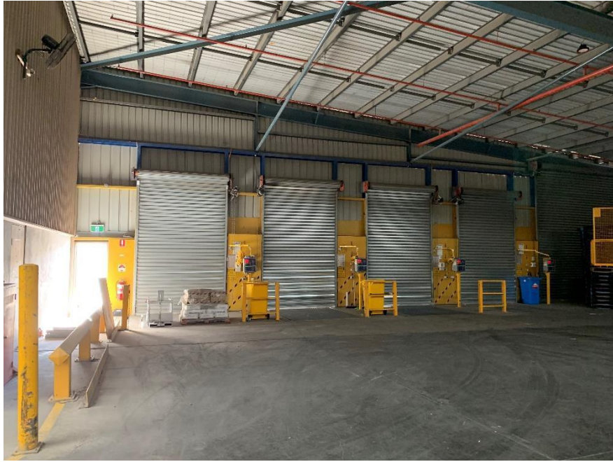
Figure 5– Internal view of Doors 3, 4, 5 and 6
