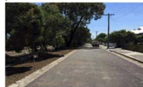
Above: Completed works in Railway Place, between Giffard to Cole Street
