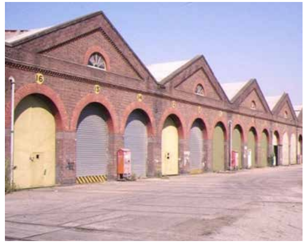
Figure 06B - Former Newport Railway Workshops (Source: Victorian Heritage Database)
