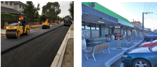
Above: works at Second Avenue, Altona North
