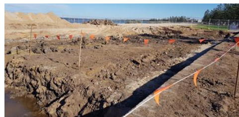
Above: slab preparation works for the shelter at McBain Street, Altona
