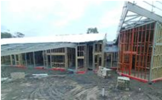
Above: Altona Early Years Hub frame works
