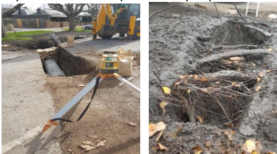
Above: Works at Electra Street, Williamstown
