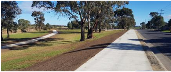
Above: completed footpath works at Carinza Reserve
