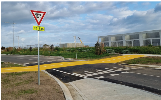
Above: New raised priority crossing for the shared path on Maddox Rd
